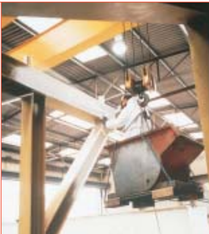
Figure 25 Manual application of Off-Site Intumescent Coatings.
