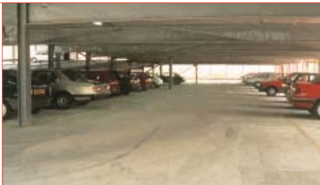
Figure 4 Steel in open deck car parks is usually unprotected.
