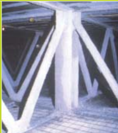
Figure 20 Board Protection Systems Photograph courtesy of Promat Ltd.
