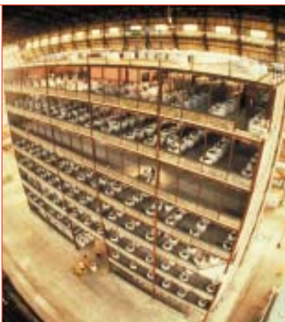
Figure 53 The Cardington Frame is a multi-storey composite structure, i.e. the floors are constructed using shallow composite slabs with profiled steel decking attached by shear connectors to downstand beams. The Level 1 Design Guidance applies only to buildings of this type.
