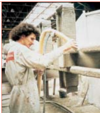
Figure 27 Off-Site Application of Spray Protection Material. Photograph courtesy of Cafco International.
